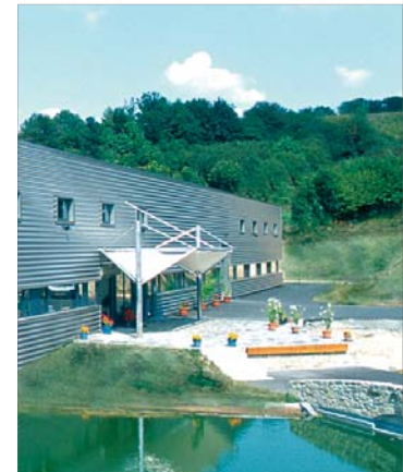
interscience R&D center and manufacturing plant
